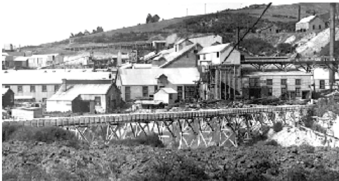
Waihi Mill (Battery) photographed from end Baker Street, c.1909
