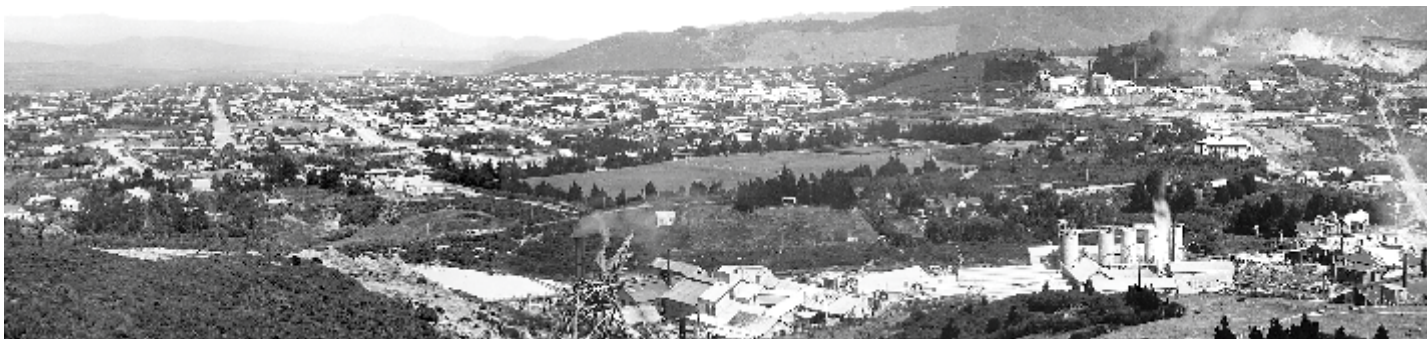
Panorama of Mill Stream Walkway area photographed from Union Hill c.1910
