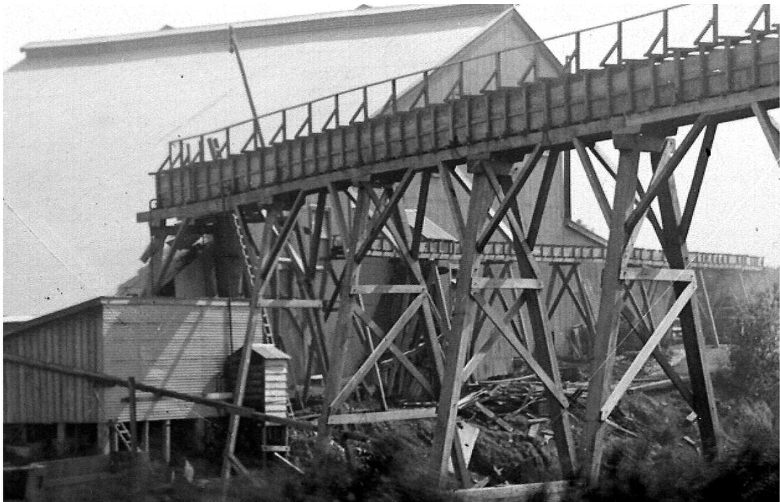
Detail. The large turbine pipe can just be made out near the left hand end of the large wooden flume. The much smaller flume in background may have been the terminus of a Mangatoetoe water race.
